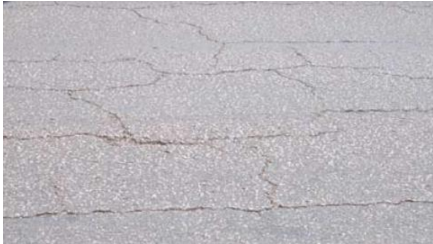
Figure 2. Block Cracking
