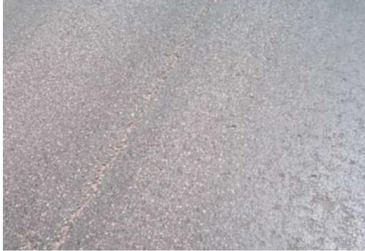
Figure 4. Longitudinal Cracking
