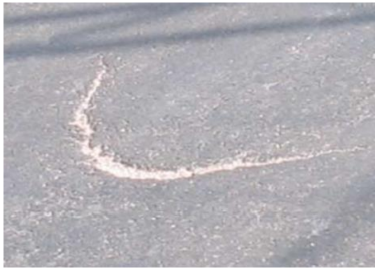
Figure 9. Slippage cracking
