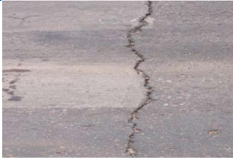
Figure 5. Transverse Cracking
