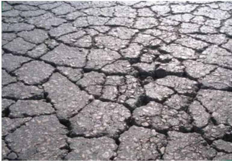
Figure 1. Crocodile cracking
