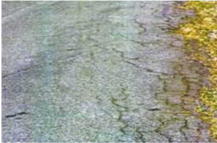
Figure 3. Edge Cracking
